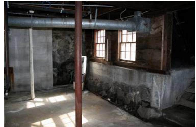
Leaking due to grading issues
