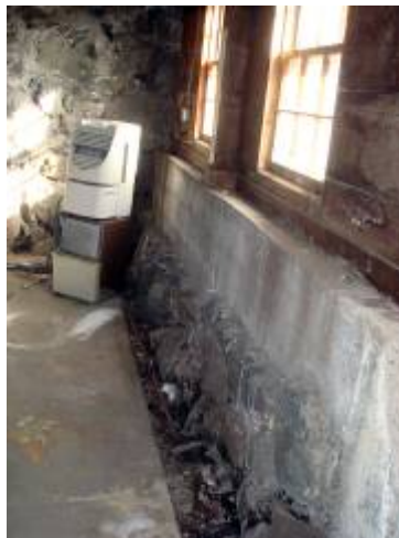
Leaking due to grading issues
